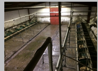
Aerial view shows the homogeneous distribution at floor and wall level.
