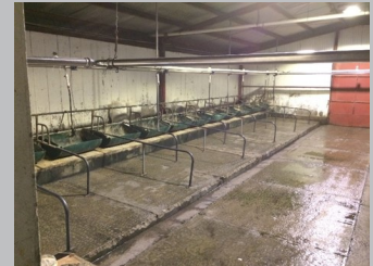
Inside right view with two 50W and 7290lm luminaires.
