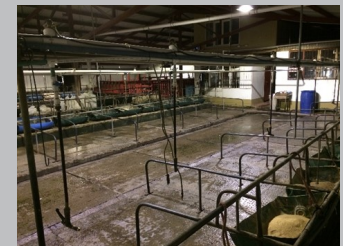
Full view, you can see the uniformity of light on both sides of the installation with the four luminaires
